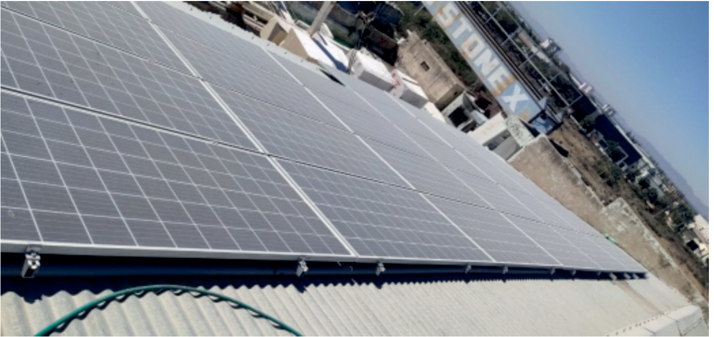
Full Rail Solutions For Metal Sheets Using L Clamps & SDS Screws
