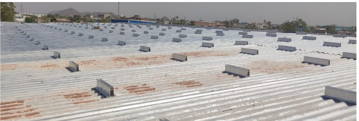
Angle Mounting For Metal ROOF North/east/west Isde Mounting For South Facing With A Tilt Angle Using Zedbox Tripod Structure
