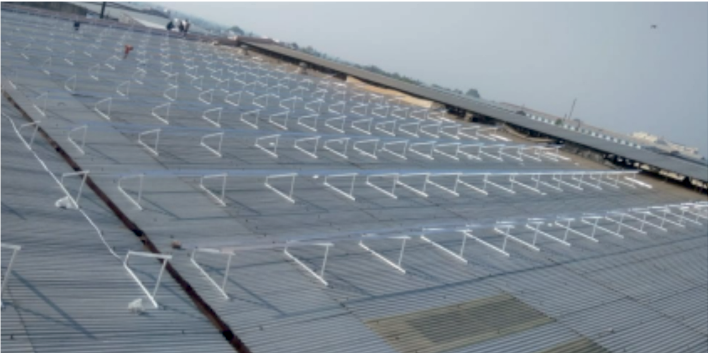
Angle Mounting For Metal ROOF North/east/west Isde Mounting For South Facing With A Tilt Angle Using Zedbox Tripod Structure
